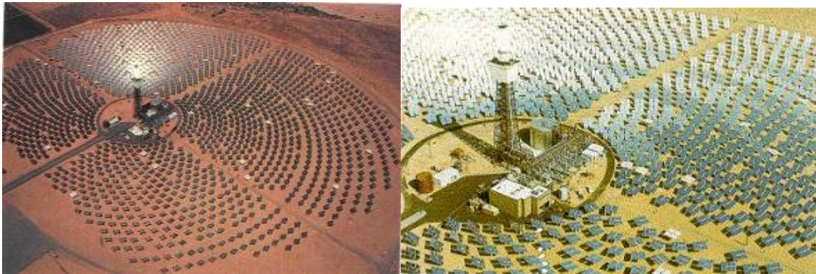
Figure 3.6. The solar central receiver (Power Tower/Solar Tower)
